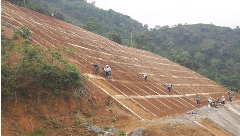
Fortified: Vetiver grass is planted on a sloppy mountain road side along Hồ Chí Minh Trails.
